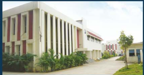
Gear Pumps Plant
