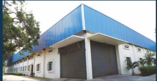
Hydraulic Valves Plant
