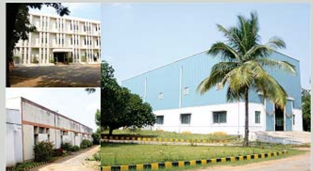
Hydraulic Cylinders & Naval Systems Plant
